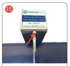
Using a wrench, rotate the stud until the guide wire is plumb and taught. (DO NOT OVER-TIGHTEN) Finalize installation using a wrench to tighten the stud to the baseplate.
