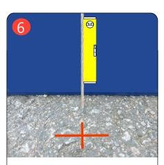
Using a level against the guide wire, pull on the guide wire until the line is plumb. Mark a line across the other 3-5/8" line as shown.
