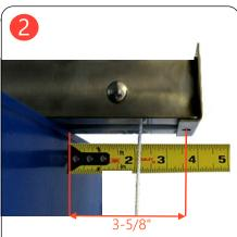
Measure from the edge of the tank to the center hole of the front plate. If you have used the Liquilevel instruction template, this measurement should be 3-5/8".
