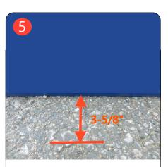
Now measure 3-5/8" out from base of tank and mark a line parallel with the tank.
