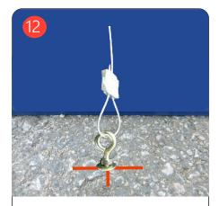
Loop the guide wire first through the fastener, then through the eyebolt and back into the fastener. Pull tight and adjust fastener accordingly. See Step-14 for more detail.
