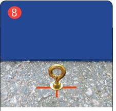
Loosen the anchor slightly by unwinding the eyebolt. Insert the M6 anchor into the hole. Using a wrench, tighten until the anchor is secured firmly into the concrete.
