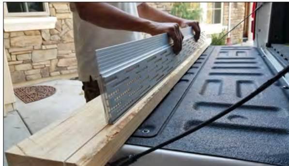
Insert Gutterglove Pro in the groove and bend downward towards yourself.
