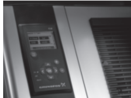
Fig. 21 Grundfos CUE control panel
